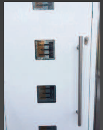
Internal view of door
